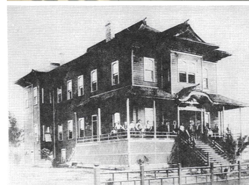
Top photo: The noble 1340 Kern Street Fresno Betsuin Temple which has served the Sangha for almost 100 years. Middle photo: Members' Farewell. Picture in front of their Betsuin Temple. Bottom photo: Original Fresno temple building 1902 - 1919.
