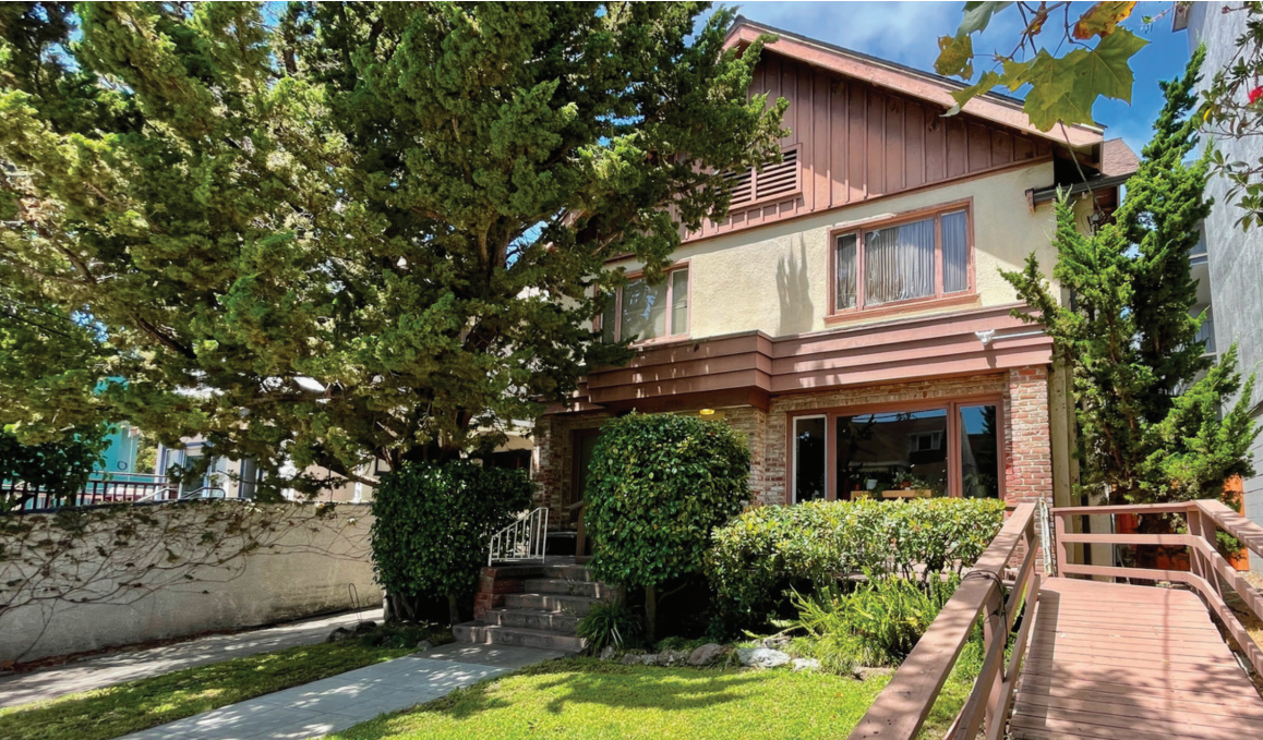
The Institute of Buddhist Studies' (IBS) Haste Street dorm is seeking donations to complete a renovation project. (Courtesy of IBS)
